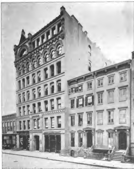
METROPOLITAN TELEPHONE AND TELEGRAPH CO., 38TH-STREET BUILDING.
